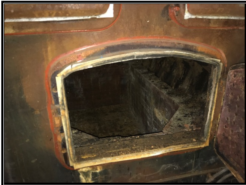
Photo 6: Non-ACM Hatch Sealant to Old Boiler - Red
