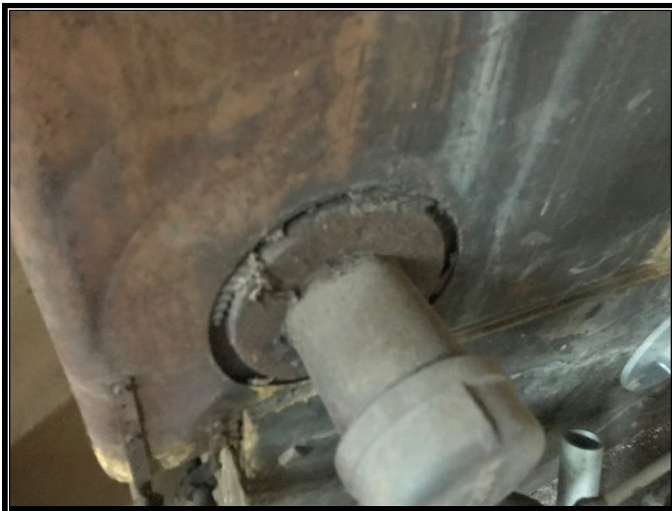
Photo 2: Confirmed ACM Rope Gasket to Old Boiler – Gray
