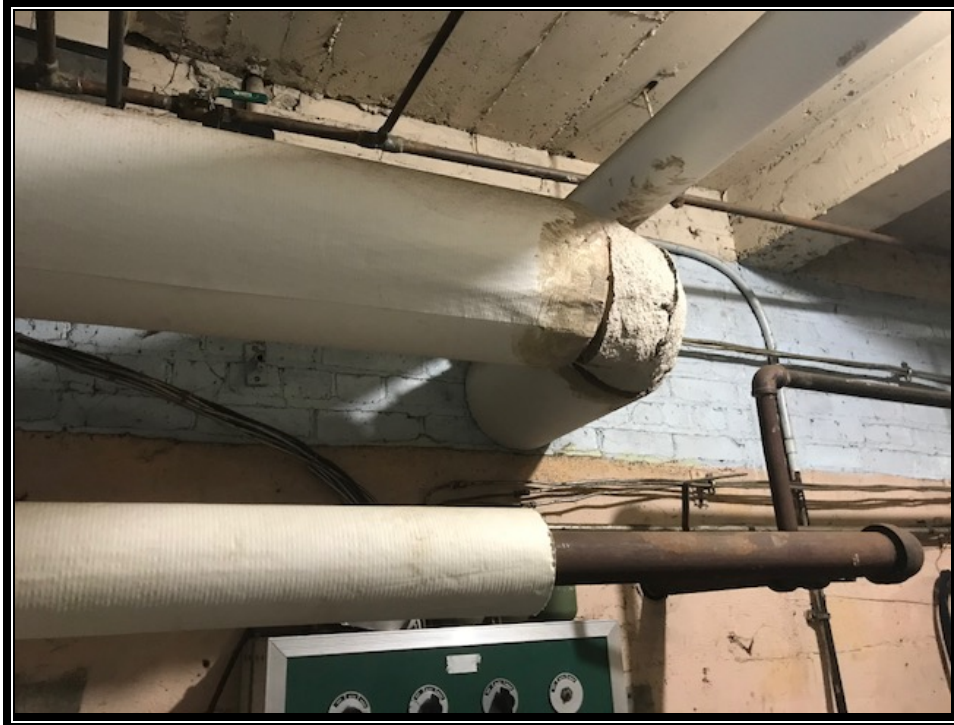
Photo 5: Non-ACM Pipe Elbow to Fiberglass Pipes – Gray
