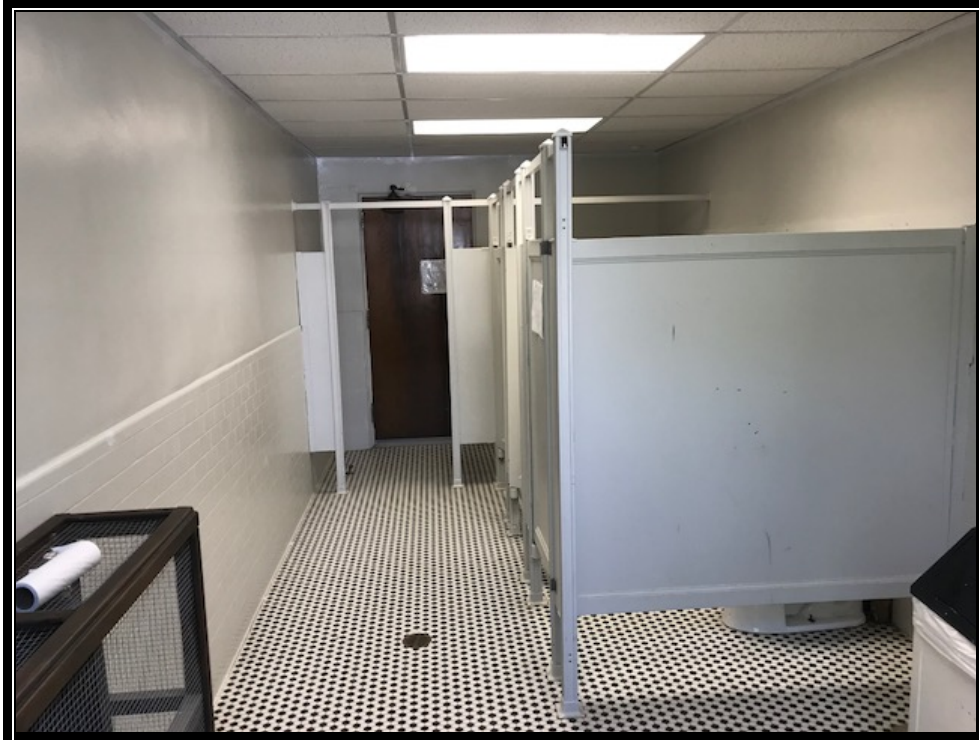
Photo 4: Non-ACM Ceramic Floor Tile Grout/Mortar – Gray, Ceramic Wall Tile Mortar – Gray, Ceramic Wall Tile Grout - White and Lead-Based Paint on Tile Wall
