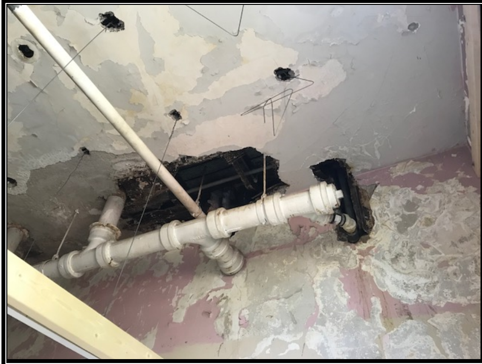
Photo 3: Non-ACM Ceiling Plaster and Wall Plaster
