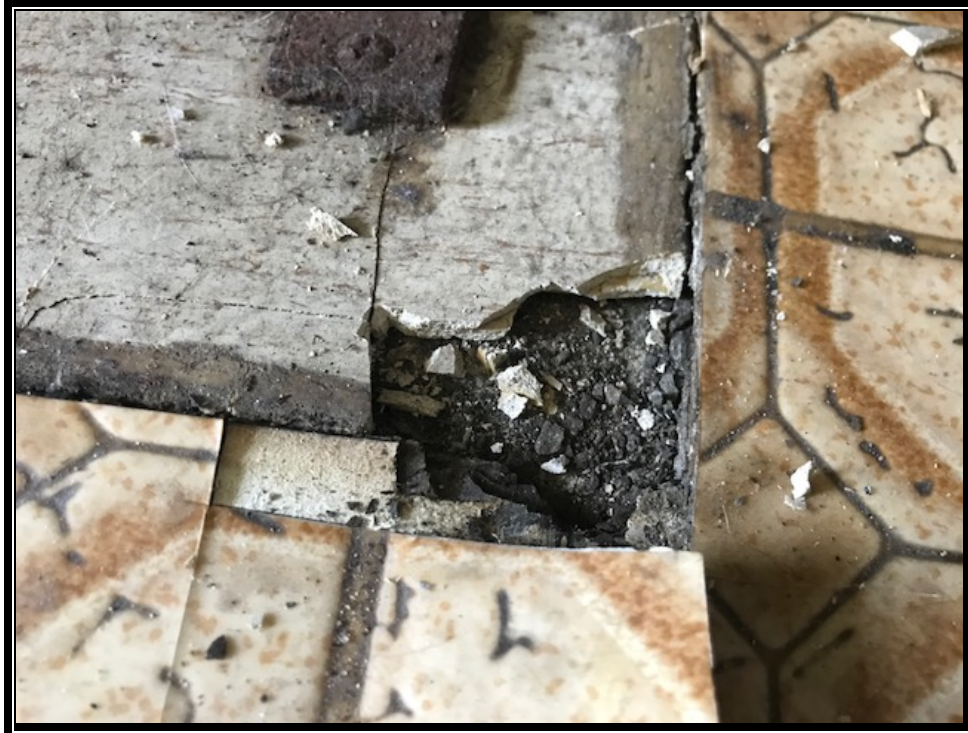
Photo 1: Confirmed ACM Mastic to Bottom Layer Floor Tile – Black, Mastic to Linoleum – Gray, and Linoleum – Brown, along with ACM Contaminated Floor Tile – Bottom Layer - White and 12'x12' Floor Tile – Top Layer – Beige
