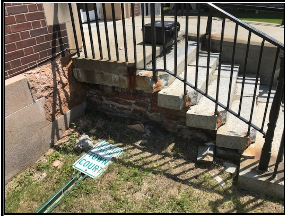
Photo 7: Non-ACM Brick Mortar to Exterior Steps at Main Entry – Gray
